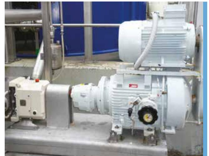
**Waste treatment plant:** open sky application on lobe pump, 11 kW unit with motor on top.
